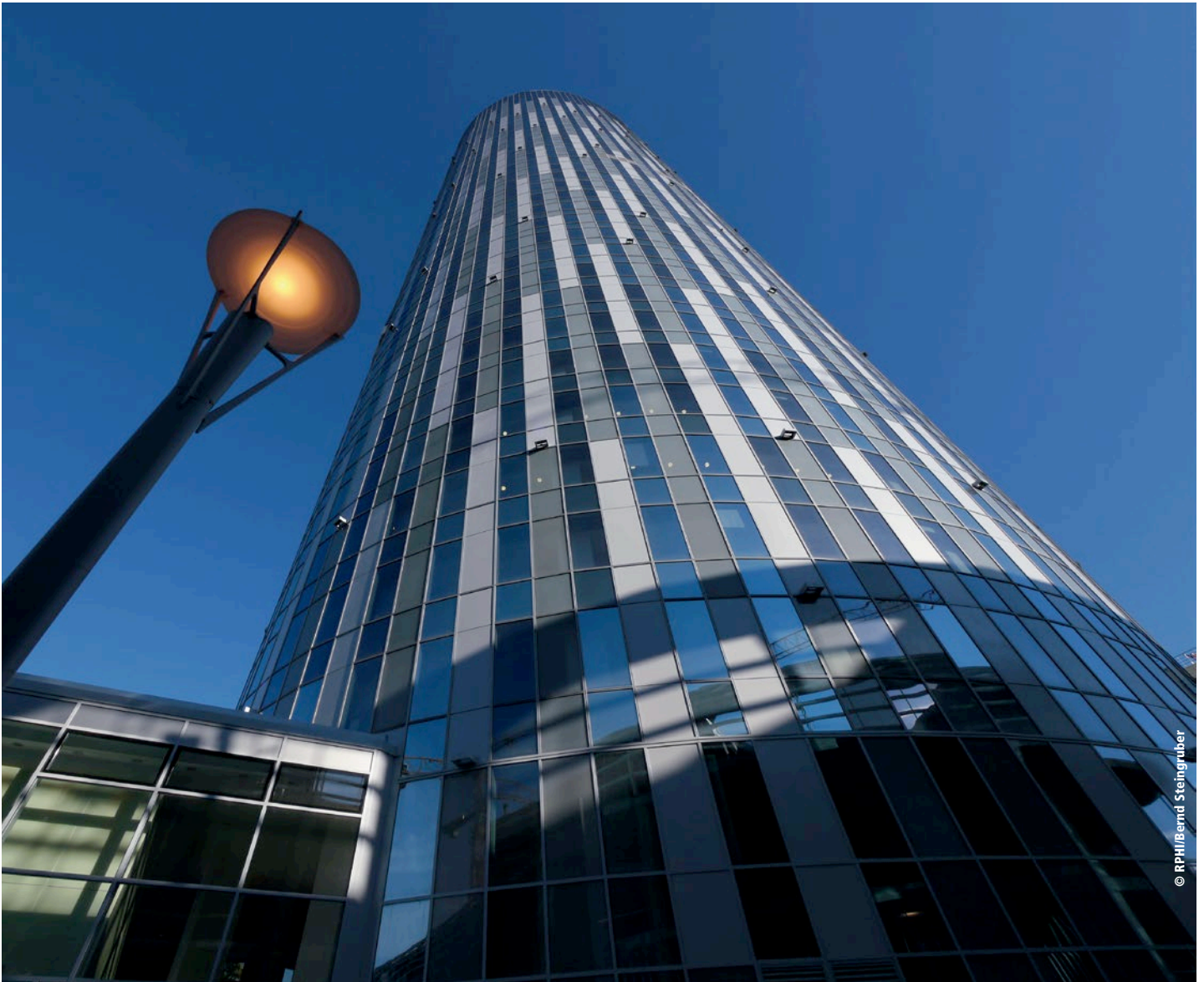
With its 37 floors and a height of 137 meters, the Sky Tower stands out in Bucharest's skyline.
