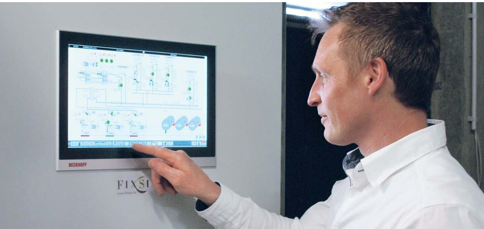
Koen Verschuere, CEO of FixSus, makes adjustments to the building management system on its widescreen multi-touch panel.
