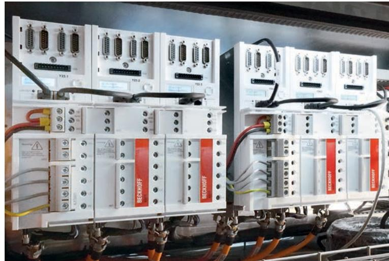
Valka uses the AX5203 EtherCAT Servo Drive to handle the motion control of the cutting robot.
