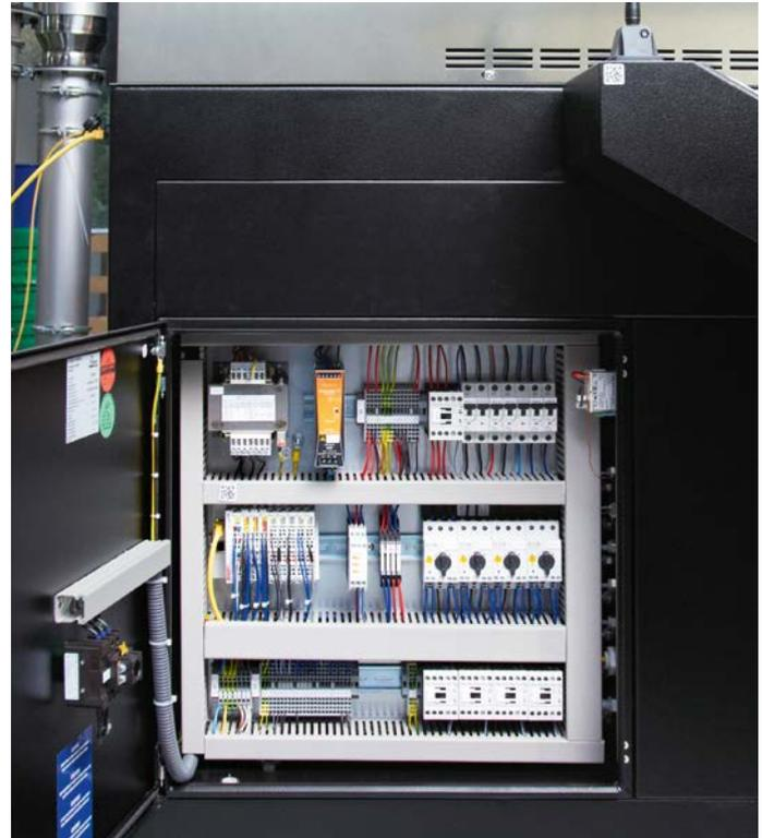
The I/O system is controlled via EtherCAT.
