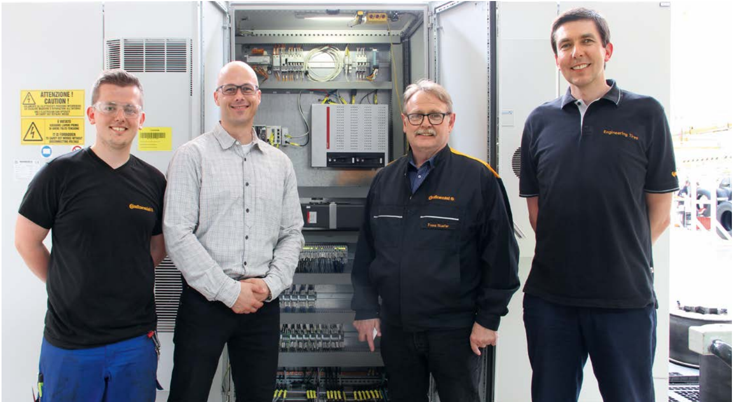
Standing in front of the many control cabinets equipped with Beckhoff control technology: Dardan Zeqiri, automation electronics technician at Continental Tires; Alexander Kruse, Key Account Manager in the Beckhoff Hannover office; Franz Stuefer, CLC plant manager; and Dr. Paul Malliband, Project Manager of Control and Drives at Continental Reifen.
