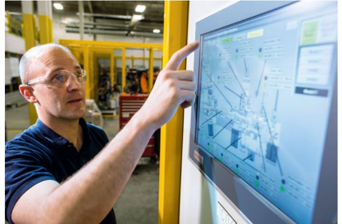
The assembly cell is controlled from a Beckhoff CP6202 Panel PC with 15-inch screen.
