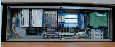
The different control elements were installed behind the skirting boards in the individual rooms, enabling full local air-conditioning, lighting and window control in line with conservation requirements.
