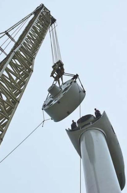
Assembly of the permanent magnet generator at the nacelle
