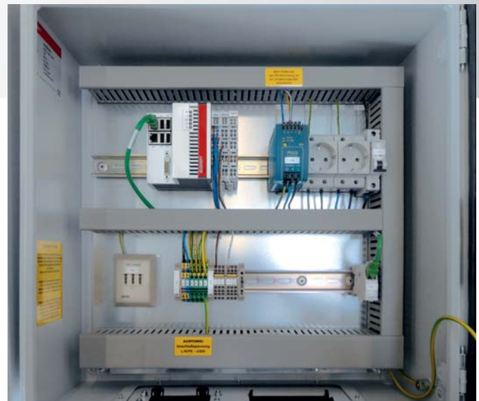
The data logger used in Aachen, Germany is approx. 40 cm in height and width, requires little space, and can be installed as an integrated solution with minimal effort.
