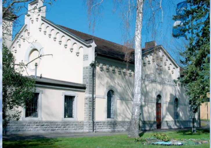
Constance Water Works was upgraded with PC-based Control technology from Beckhoff. This results in higher operator comfort and improved security of supply.
