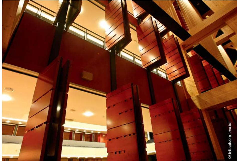
The Sibelius Hall is flanked by wall-high echo chambers, which are equipped with 188 mobile acoustic doors. A Beckhoff Embedded PC from the CX series controls the positions of the acoustic doors via the KL2612 relay terminals. The reverberation time can be precisely adjusted according to the resonance effect desired by the musicians.
