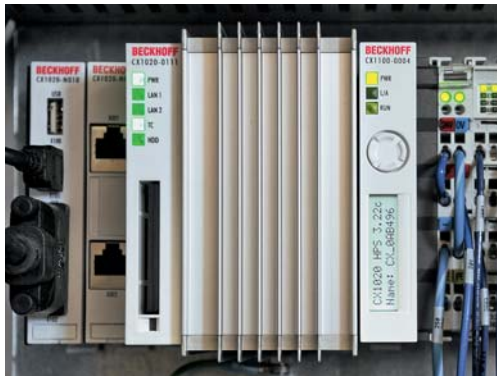
Beckhoff CX1020 Embedded PCs with the TwinCAT PLC automation software and EtherCAT I/Os are used as the control platform for the check weighers from Friesen's.
