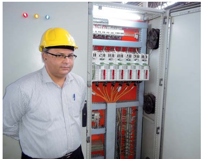
Maneck E. Behramkamdin presents the control cabinet space, which is optimally used by the compact AX5203 2-channel servo drive with One Cable Technology (OCT).
