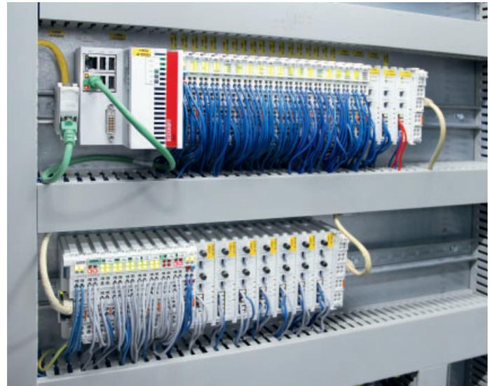
Eight CX5020 Embedded PCs are used as floor controllers in the ZVE.
