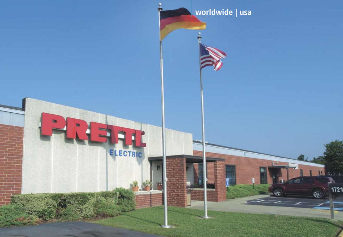
The US facility of Prettl Electric in Greenville, South Carolina.
