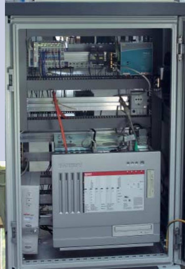
Control station of the production line, consisting of a control cabinet PC C6140 and a Beckhoff Control Panel.
