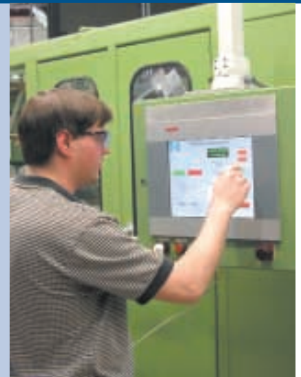
Wirsbo retrofitted several pieces of equipment with Beckhoff IPC and touch screens.
