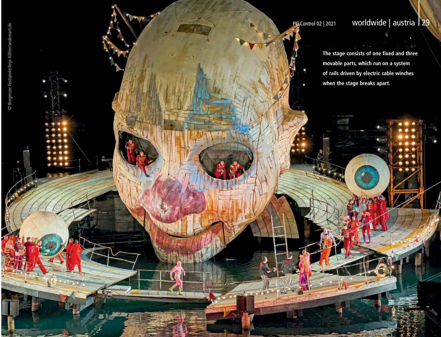
The stage consists of one fixed and three movable parts, which run on a system of rails driven by electric cable winches when the stage breaks apart.
