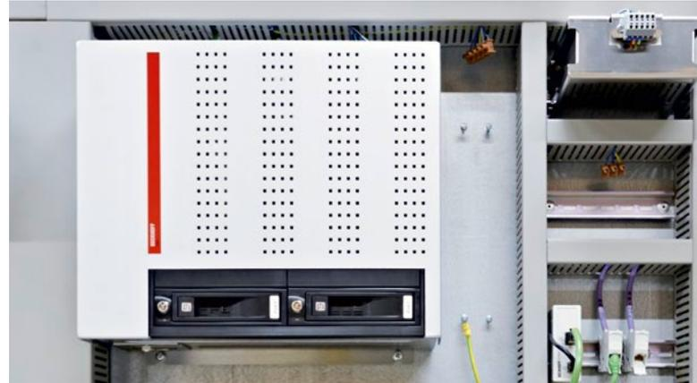
A C6650 control cabinet Industrial PC with multi-core processor is used for higher-level control and monitoring of the entire Lisocore® production plant.
