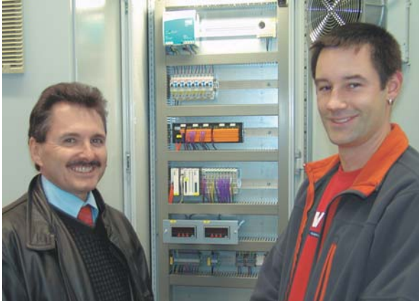
André Duss (right), from BSR Automation AG, and Robert Urech, from the Swiss branch of Beckhoff Automation AG, in front of the control cabinet of the MGB test rig
