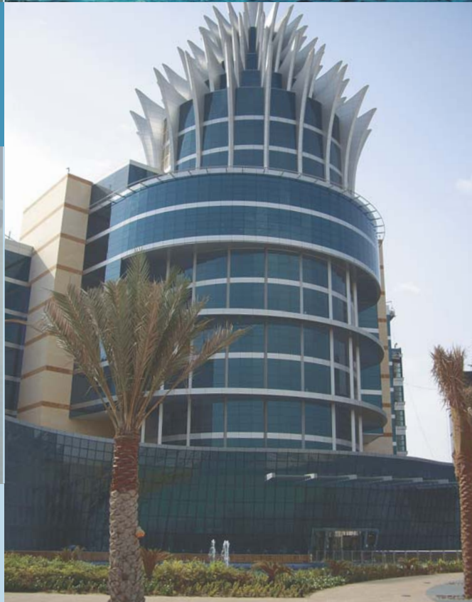
Beckhoff office in Dubai
