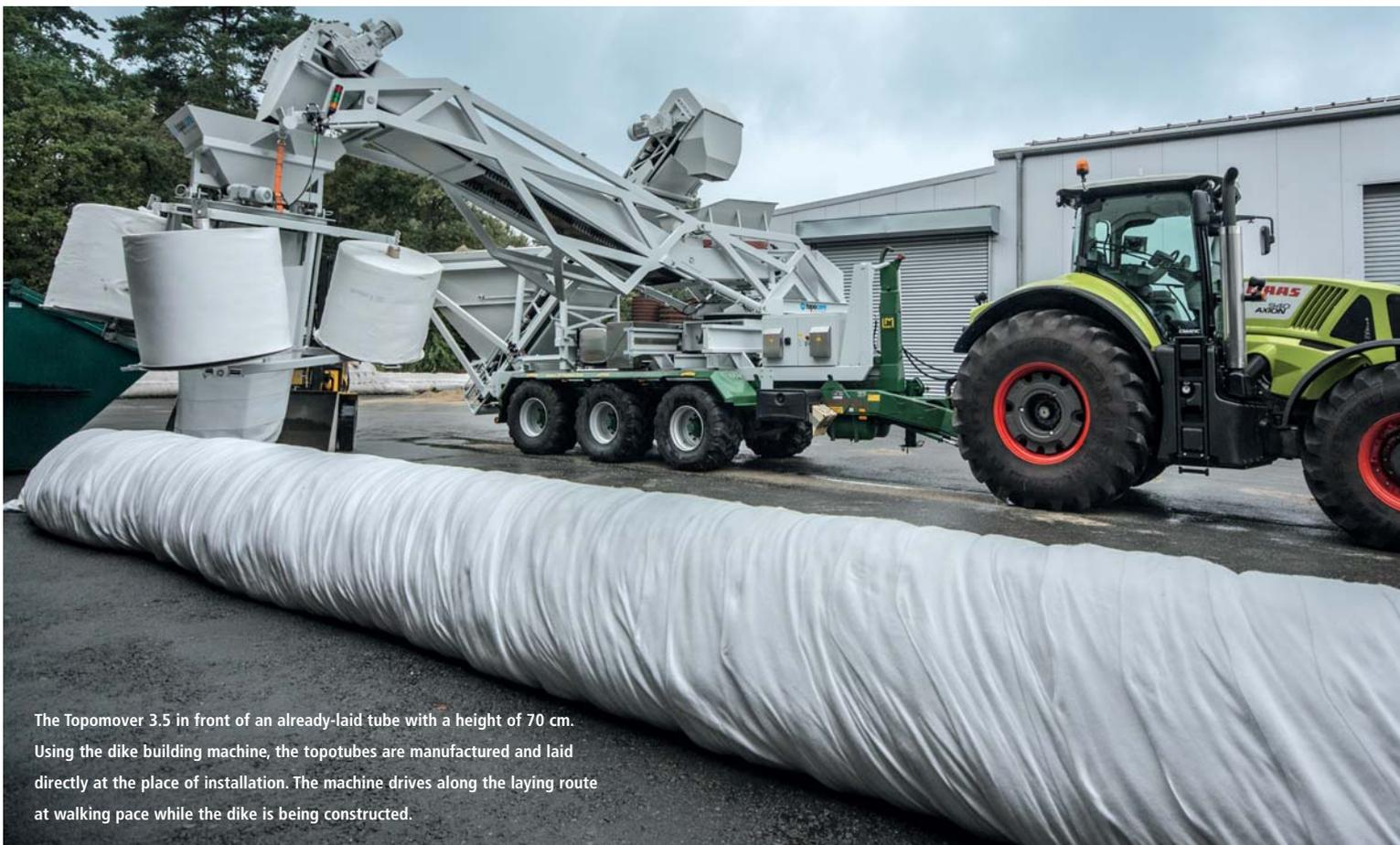
The Topomover 3.5 in front of an already-laid tube with a height of 70 cm. Using the dike building machine, the topotubes are manufactured and laid directly at the place of installation. The machine drives along the laying route at walking pace while the dike is being constructed.
