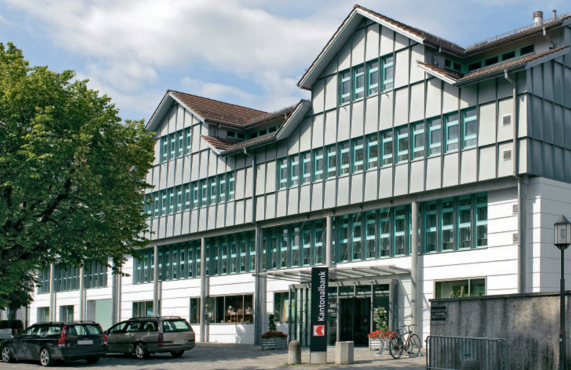
Head office of Appenzeller Kantonalbank in Appenzell. The extension (rear, left) subdivides the building complex into three architecturally equivalent parts. At the same time, the existing building was extensively refurbished.
