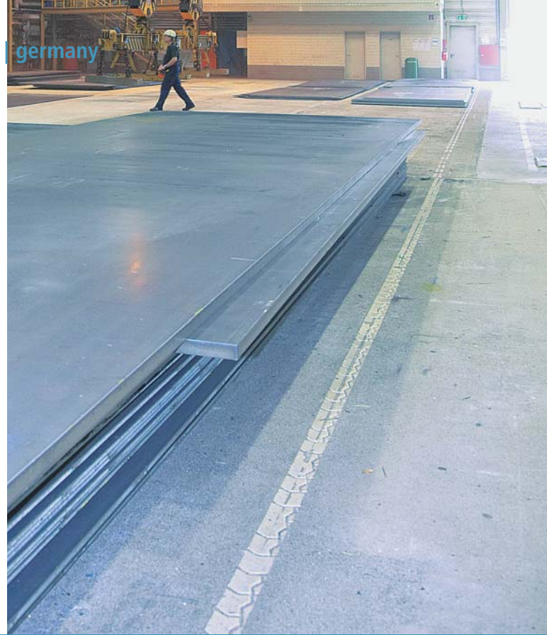
New cutting hall with three flame cutting machines from Messer Cutting & Welding GmbH
