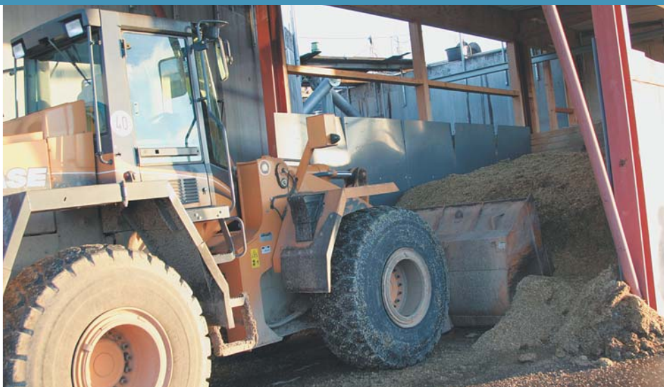
The biogas plant has an output of 500 kW. It is fueled with biomass such as corn silage or liquid manure.
