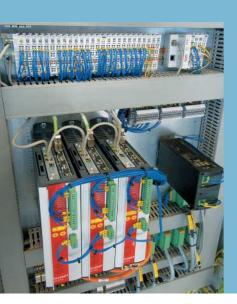
I/O and drives are integrated in the control system via EtherCAT for high-performance positioning.
