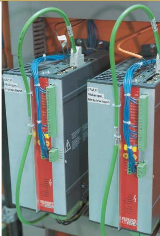
trol system was replaced. Continental's control engineers chose PC-based controllers from Beckhoff as their platform. Four C6130 Control Cabinet PCs were used, each with a 15 inch CP7002 or CP7032 Control Panel. Two of the four IPC/Panel combinations are used for recipe management and visualization, a further combination controls the cutting machine, and the fourth one deals with color marking.
