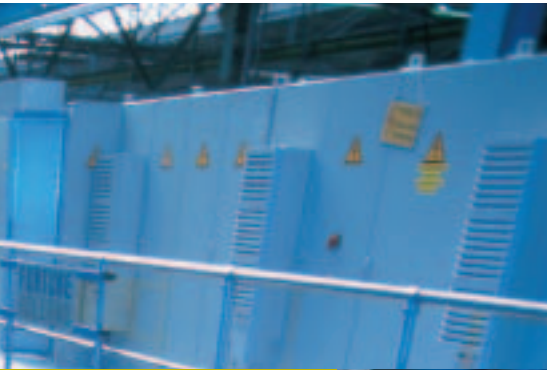
Overview of the Hayes-Lemmerz wheel rim line consisting of reeling, welding and profiling units.
